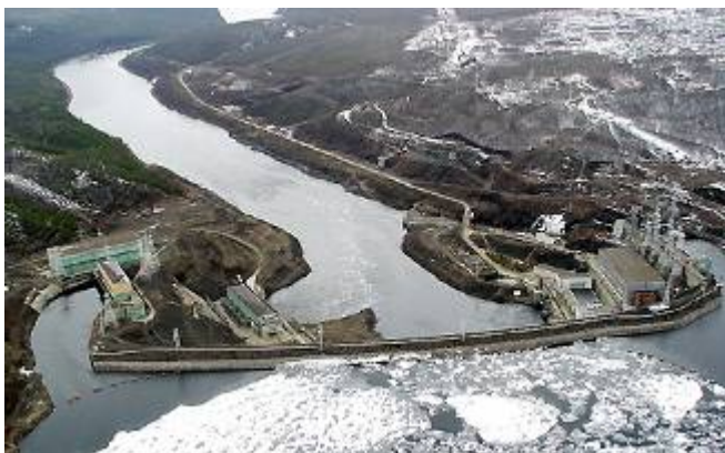
Figure 47: The Vilyui HPP
